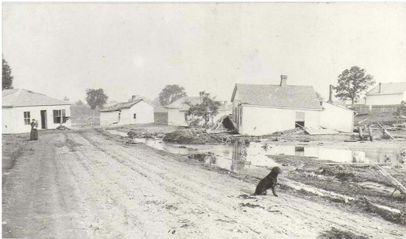
Figure 3. Flood damage on Blackfriars Street looking west, near Wharncliffe Road. (Source: Archives and Regional Collections Centre, UWO)
